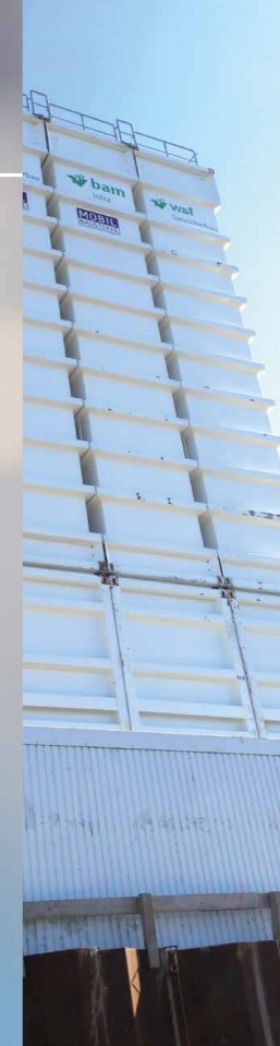
Concrete batching plants
