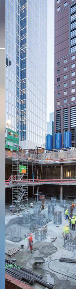
Special foundation engineering
